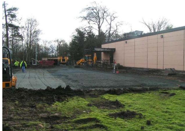
Edinburgh: laying foundations for new plant room
